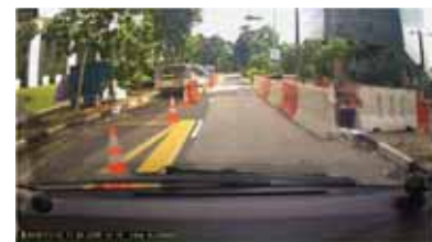
Road construction and jay walking
