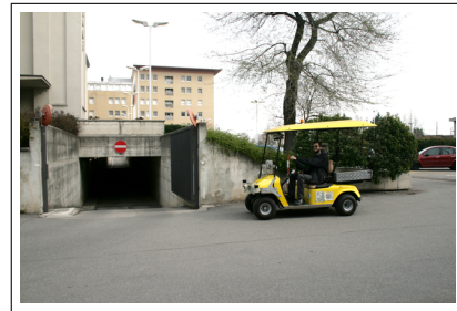
Fig. 13. The ramp from the underground garage to the outdoor park, picture taken from the outdoor park.
