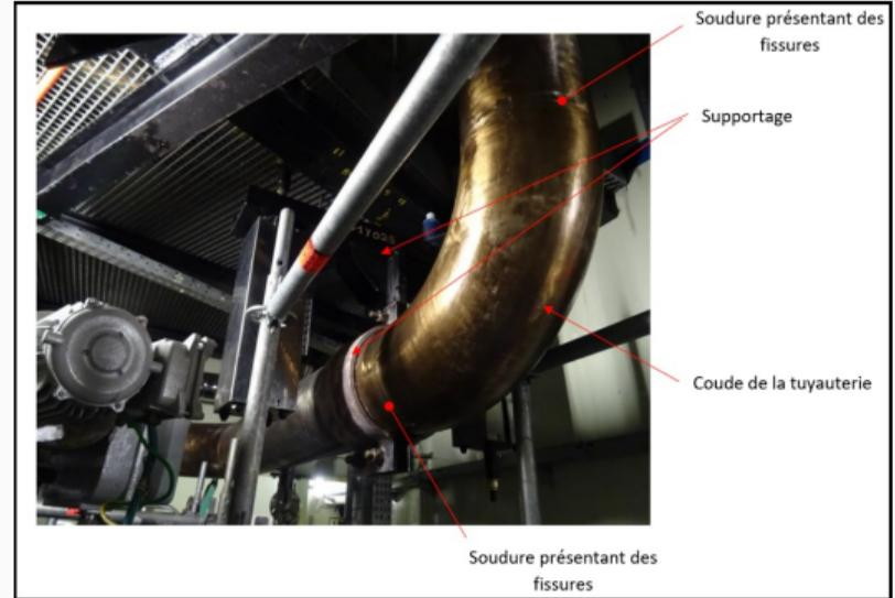
Stress corrosion cracking spotted by *ultrasounds*.
