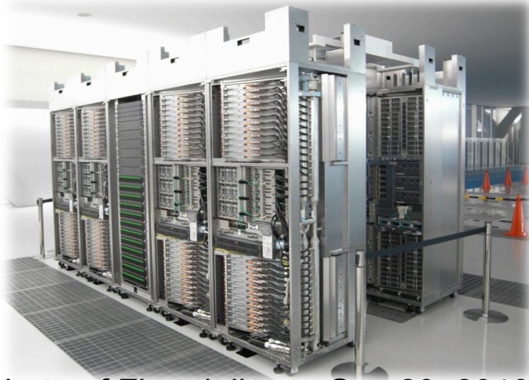
Photo of First delivery, Sep 28, 2010
